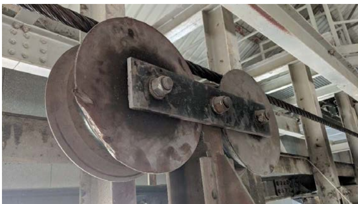
Roller Damages seriously damage the rope
