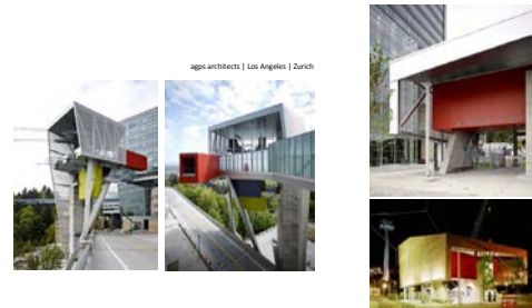
Dar. 12 agps. architecture | Aerial Tram | Portland 2007
