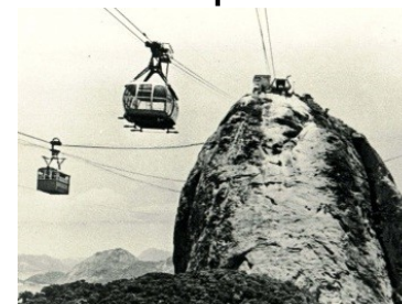
Upgrade – The New Cable Car
