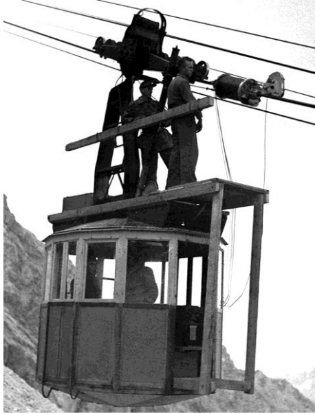
Figure 2: DC excited rope inspection on an ancient Bleichert jig-back, Zugspitze 1950s.
