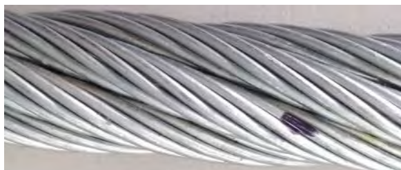
Figure 4-13: Single wire break in strand touching zone
