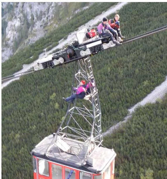
Figure 3-10: Visual inspection of track ropes on a special platform to sit or lie down
