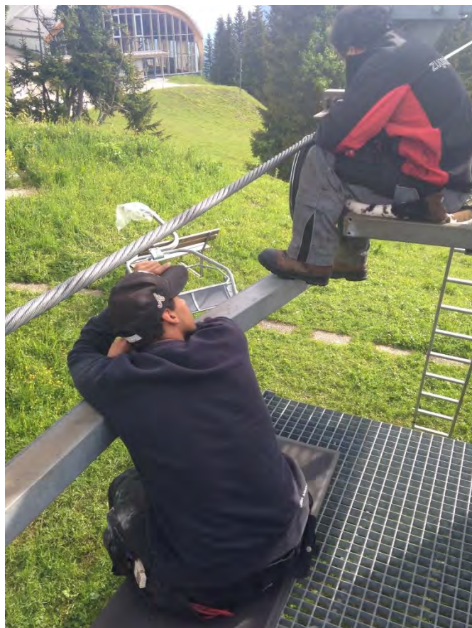
Figure 4-31: Workplace environment second installation top station
