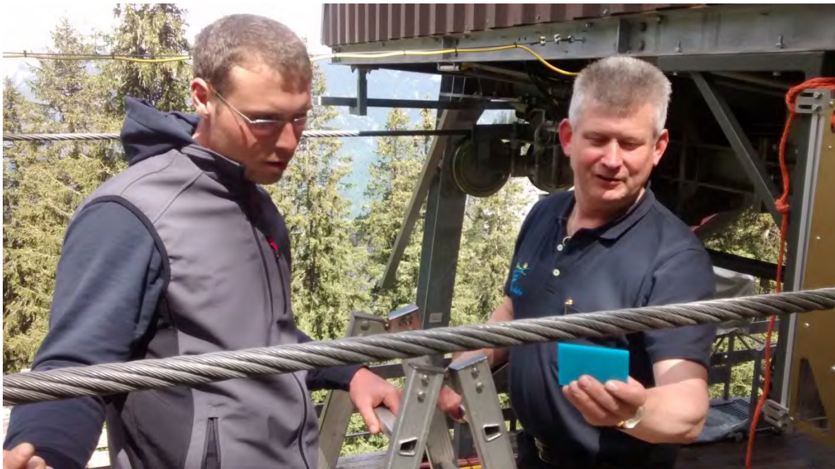
Figure 5-22: Inspection with hand mirror
