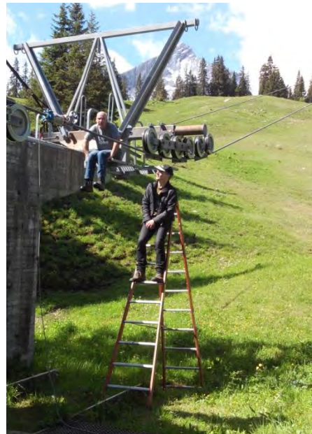
Figure 3-2: Visual inspection on a ladder and a small platform
