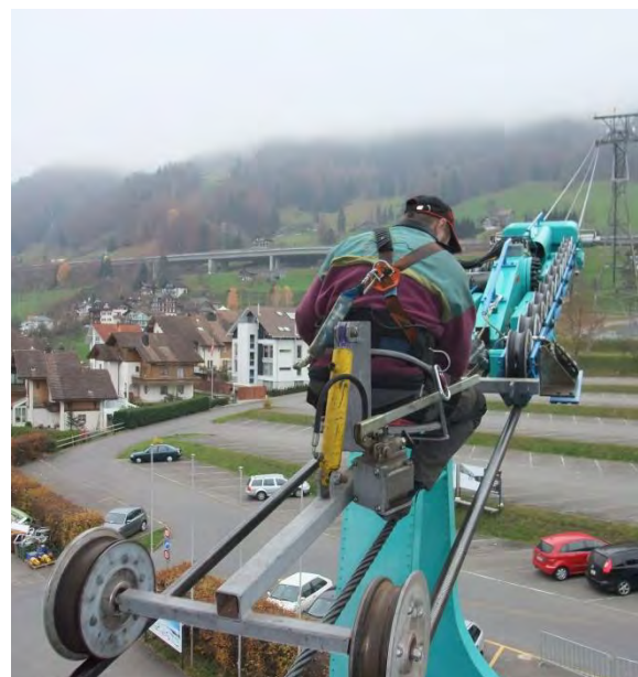
Figure 3-11: Visual inspection of track ropes with a special seat
