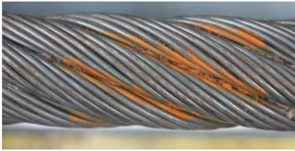
Figure 4-21: Corrosion in strand touching zone
