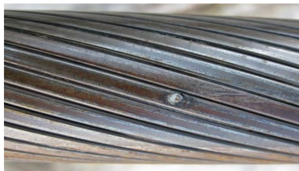
Figure 2-13: Lightning strike at locked coil rope
