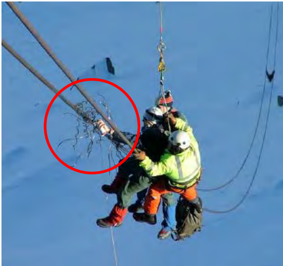
Figure 2-8: Track rope damage [6]
