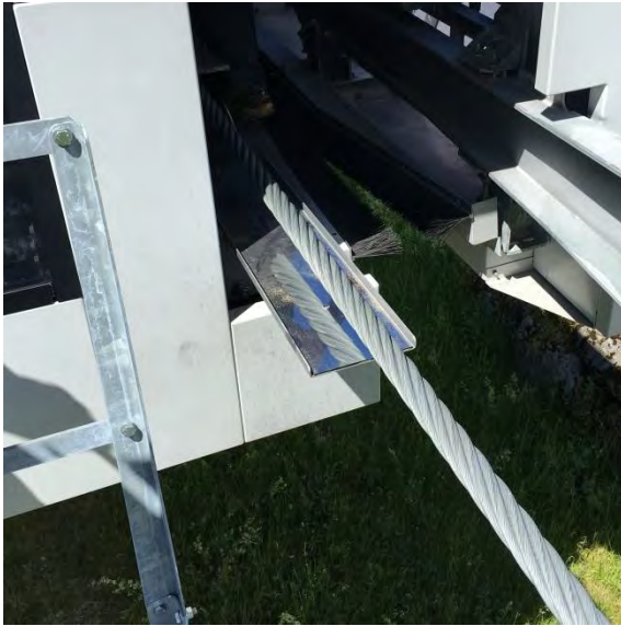
Figure 3-12: Mirror at a standardized modular station for monocable aerial ropeways (View from the outside)
