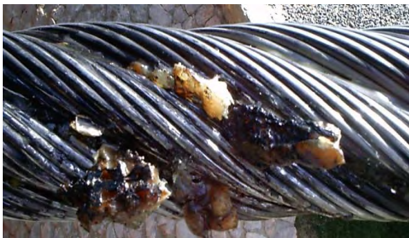
Figure 2-12: Lightning strike with huge damage at strand rope
