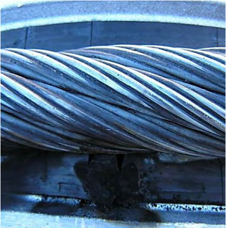
Figure 2-5: Damage by current flow
