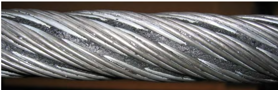
Figure 6-14: Dirt in strand touching zone - hard to inspect
