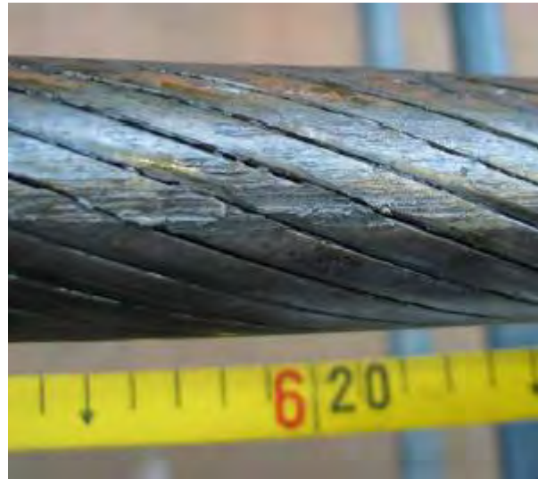
Figure 2-9: Track rope damage – detail [6]
