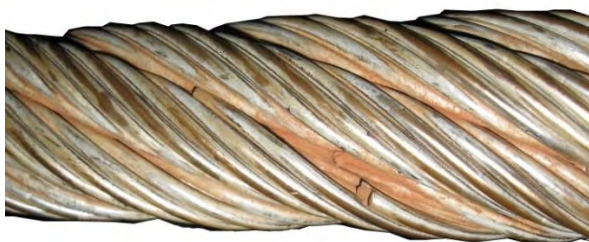
Figure 4-17: Strand touching zone corrosion (with wire breaks)
