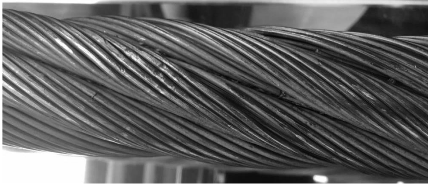
Figure 5-25: Damage which could be found during the inspection
