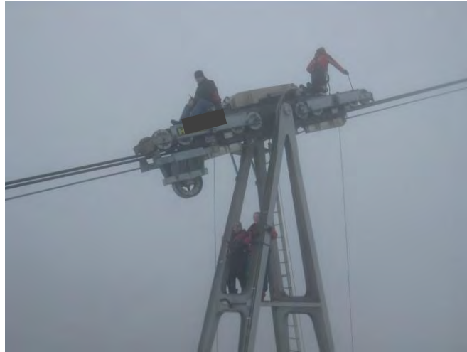
Figure 3-3: Fog during track rope inspection
