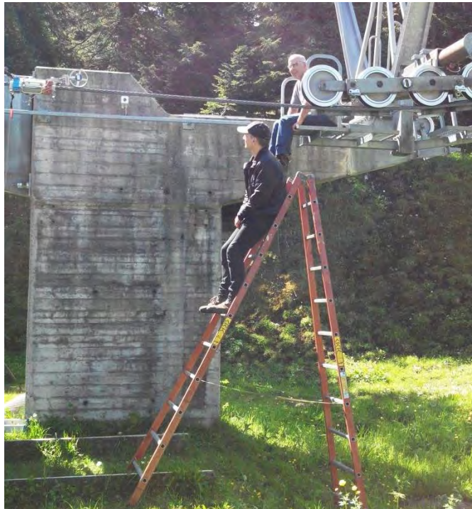
Figure 4-30: Workplace environment second installation bottom station
