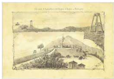
1889 Material ropeway Valestra – Oca (Tree trunks – Length 5 km)
