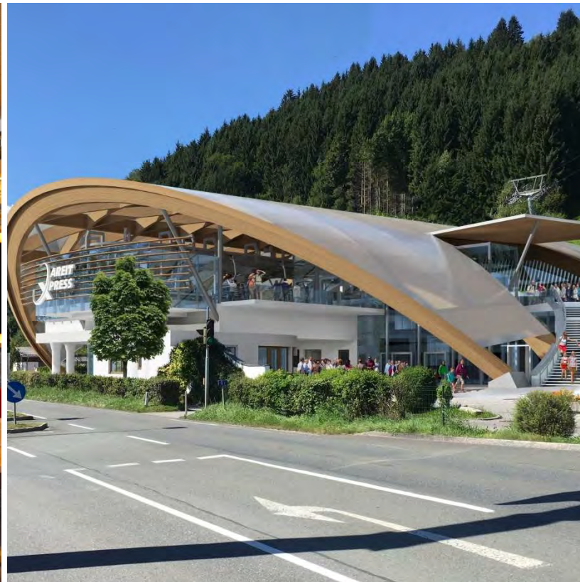
Engine heat areitXpress Energy saving of 84,000 kWh/a
