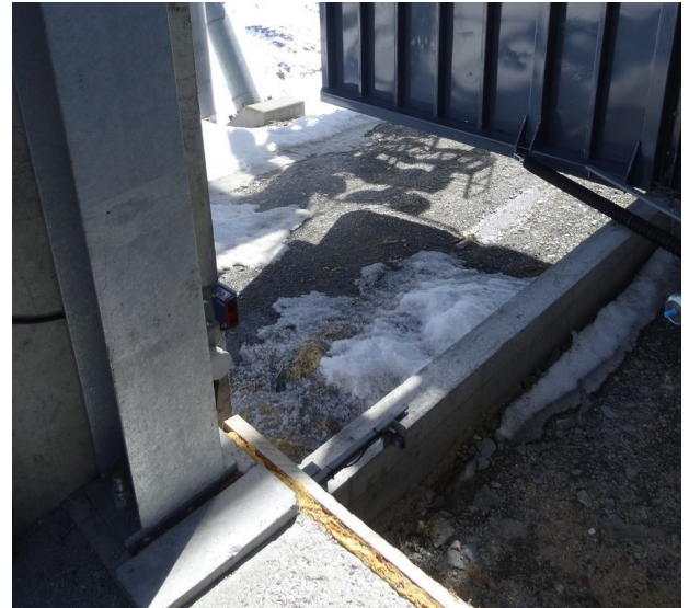
On these photos from the top station of jigback-operated Funitel Trois Vallées (ex-Bouquetin), we can see such presence detectors in the pit and on the edge of the platform.
