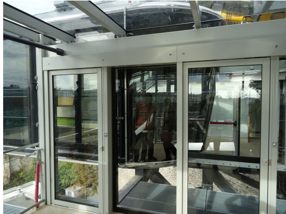
→ TPH Brest, Jean Moulin station
