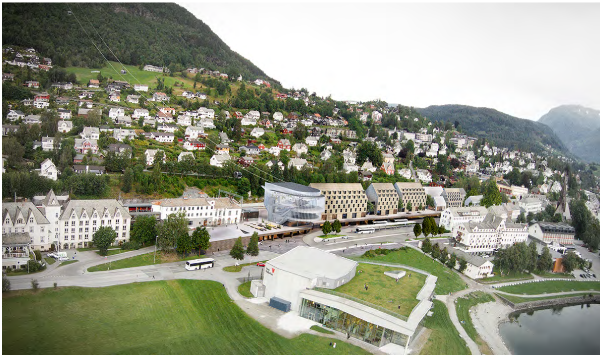
Figure 2 Overview of the lower station area, railway station and hotels.
