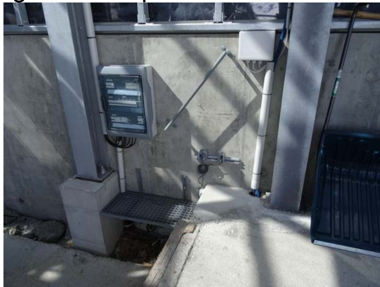
→ FT Trois Vallées – Bouquetin : bottom pit and platform detection cells
