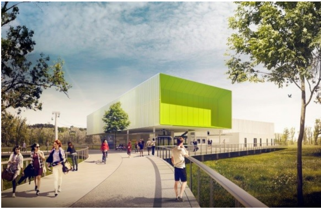
Station Oncopole / Oncopole Station © Groupement POMA
