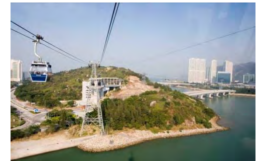
Cable car technologies
