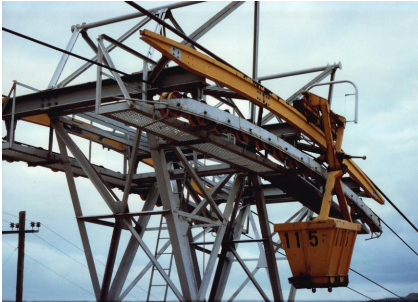
Rio Branco tower with fixed saddle and “high” roller battery
