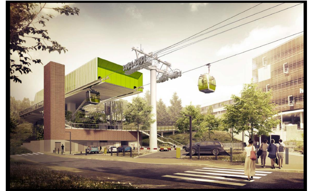
Proiet Monocâble / Single-cable project © POMA
