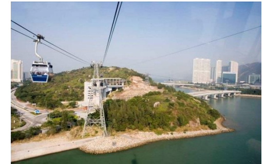
Cable car technologies
