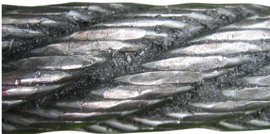
Abrasion or crush of the outer wires of several strands
