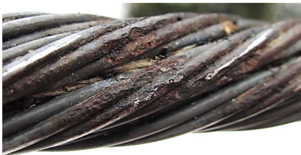
Wire breaks due to corrosion
