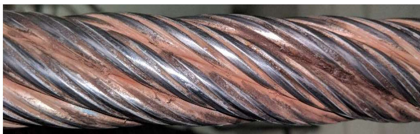
Corrosion induced by friction between touching strands
