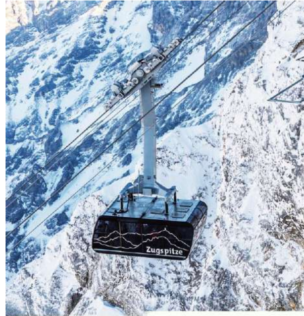
120 ATW-Zugspitze Highest steel lattice tower (127 m), largest vertical rise (1,945 m) and longest rope span (3.213 m) of a ropeway worldwide
