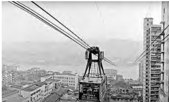
Chongqing cableway in China, retired after 20 yrs of operation, should be now running again
