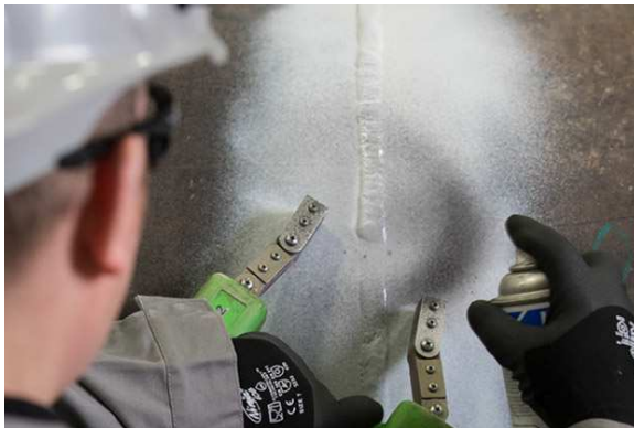
Magnetic Particle Testing
