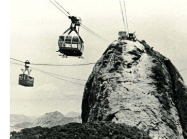
Upgrade – The New Cable Car
