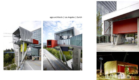
Dar. 12 agps. architecture | Aerial Tram | Portland 2007
